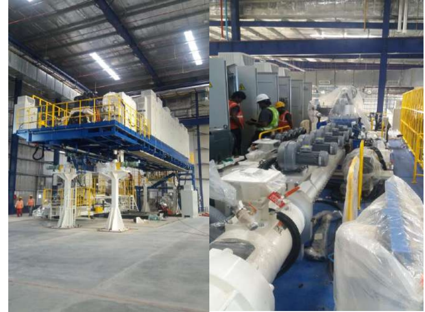
PLASTIC OMNIUM (GJ) Job Type :Installation of Blow moulding machine
